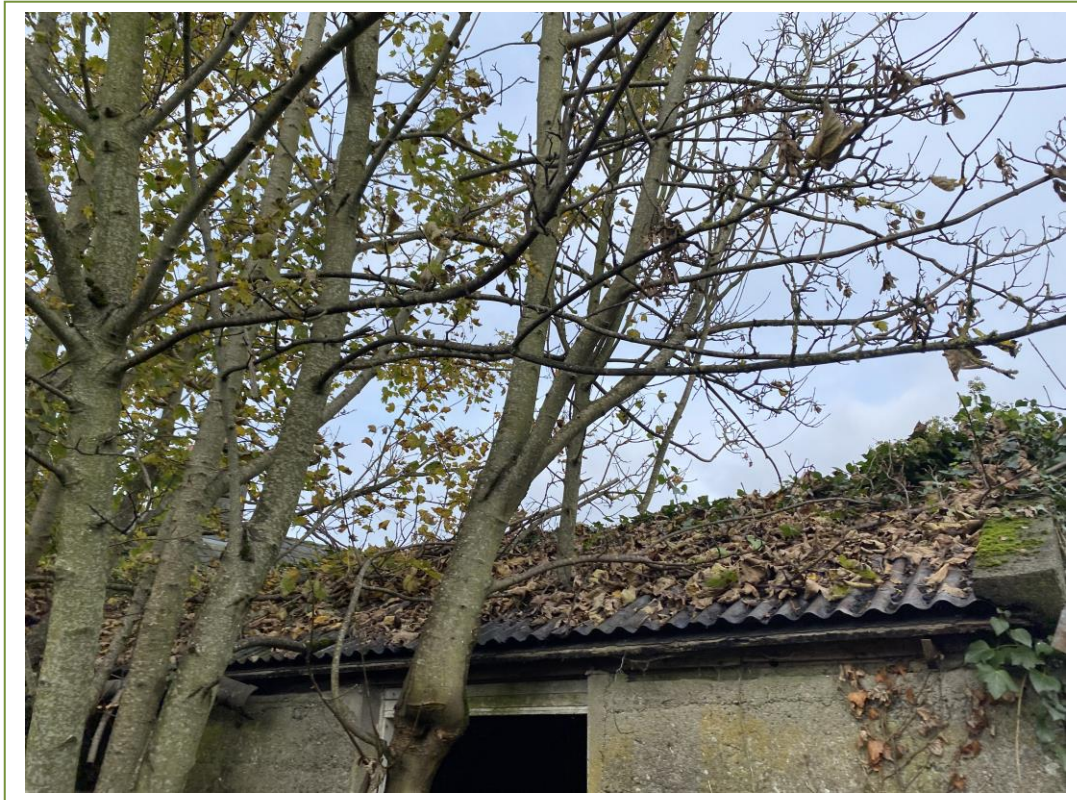
Metal cladding on the roof of the rear shed
