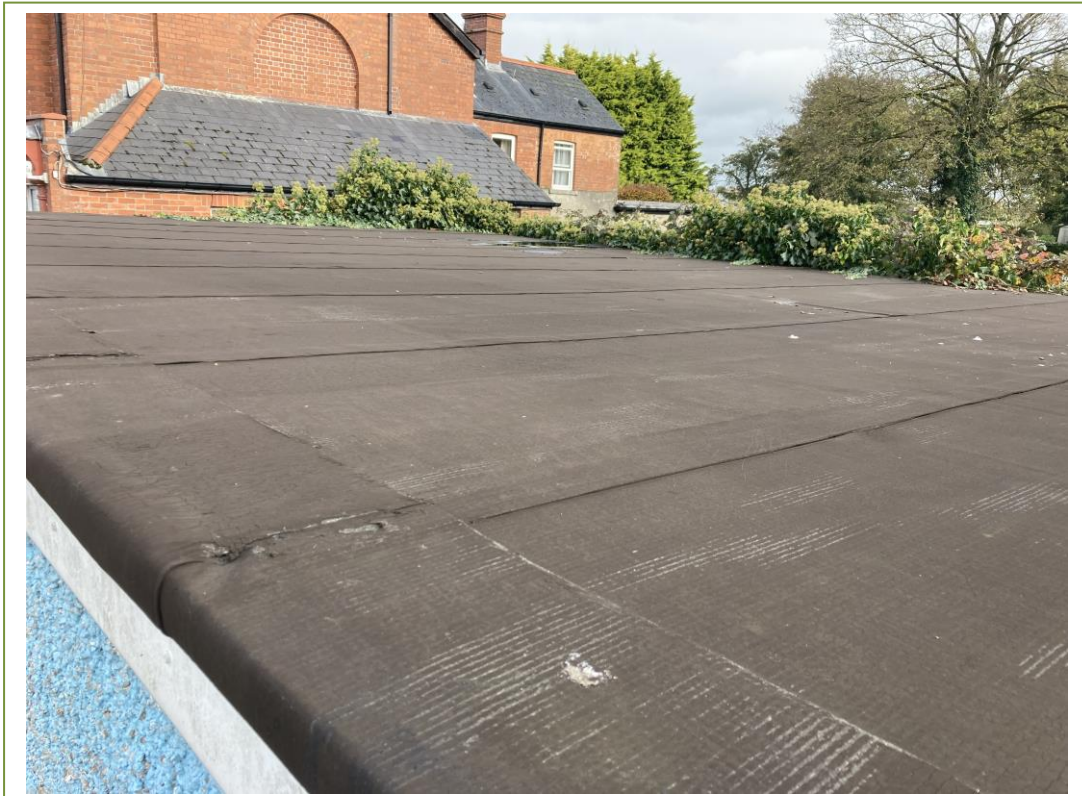
Felt sampled from the roof of the garage
