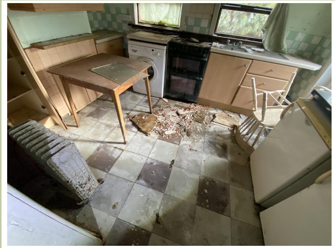
Vinyl floor tile sampled throughout
