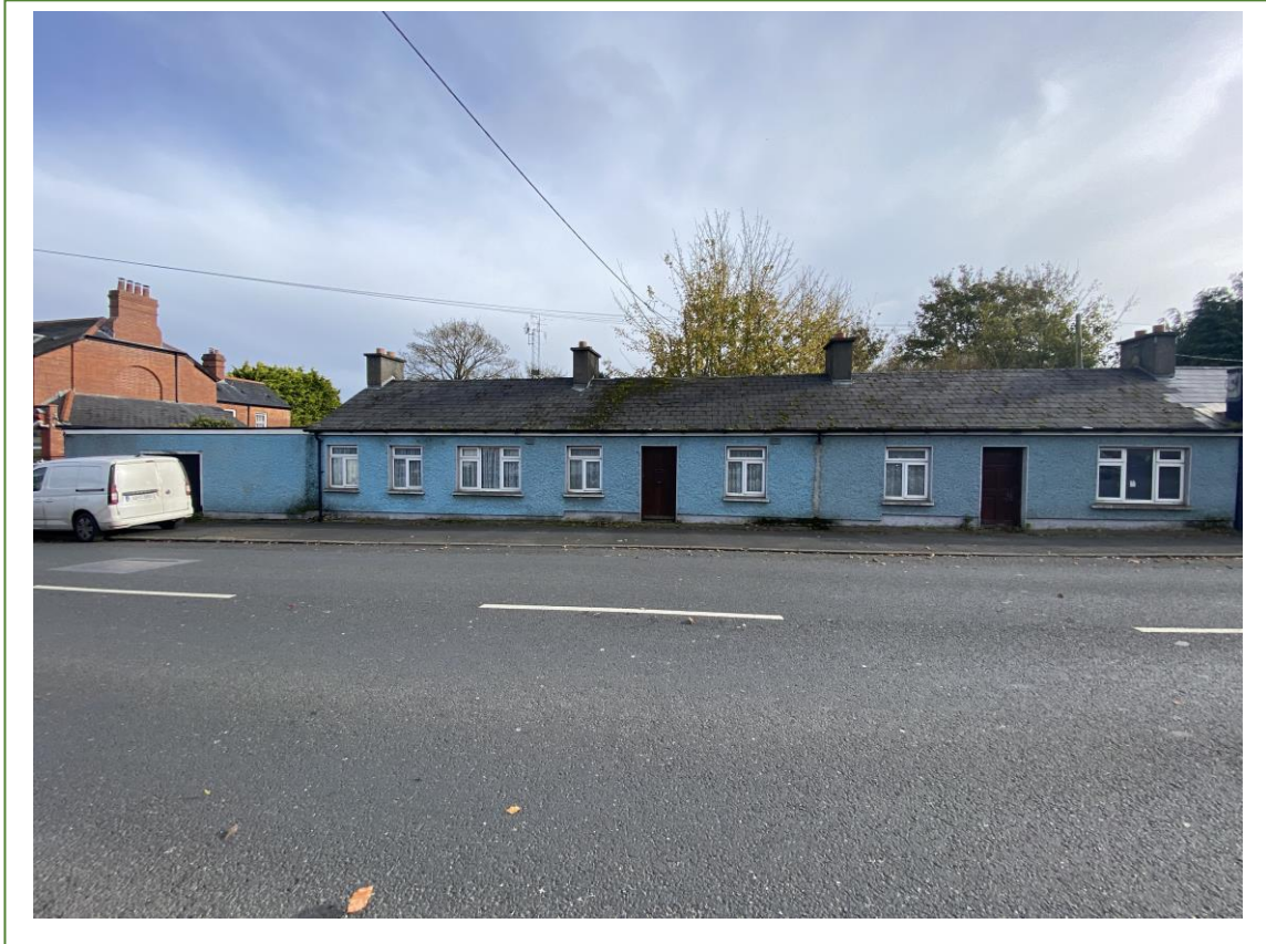
Derelict Houses Site, Station Road, Kildare Town, Co. Kildare
