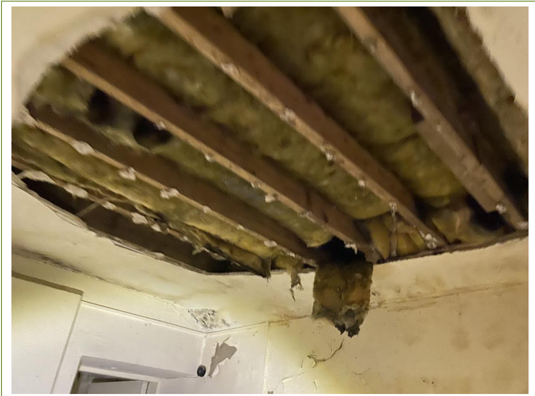
Plasterboard ceilings & fiberglass insulation
